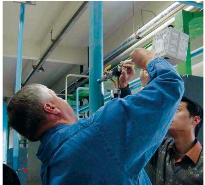
*With Kaeser's ADA, data logging with highly accurate sensors are attached to the system to monitor the compressed air usage*
